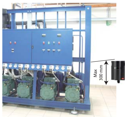
Per gas: R22 - R134a - R404a - R407a - R407c - R410A h max 300 mm
