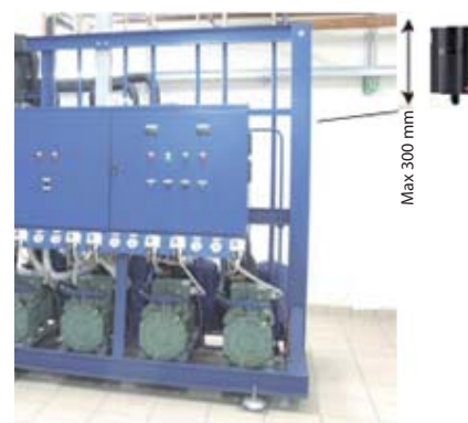
Per gas: NH 3 - ETHYLENE h max 300 mm from ceiling
